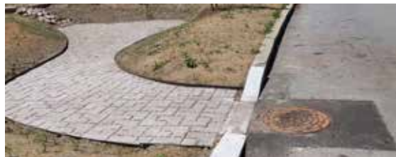
Located near the Seal House in Roger Williams Park, stormwater runoff is directed to flow into this infiltration basin. The first part of the structure, the cobblestone-like forebay, is a landing spot for the runoff to slow down and temporarily pool up.
