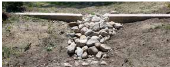
The dam-like structure that stops the water and allows the sediment to drop is known as a weir.
