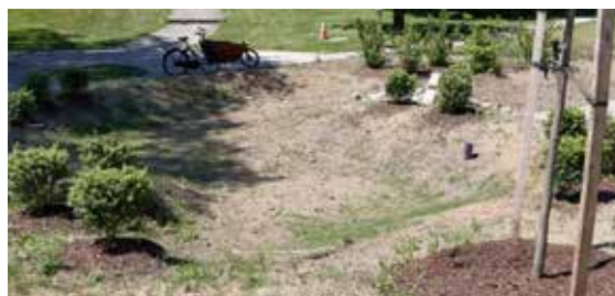
An infiltration basin is a shallow basin of modified soils and native grasses where stormwater remains for 24 to 48 hours after flowing over the weir. It is slowly absorbed into the ground, removing contaminants from the water.
