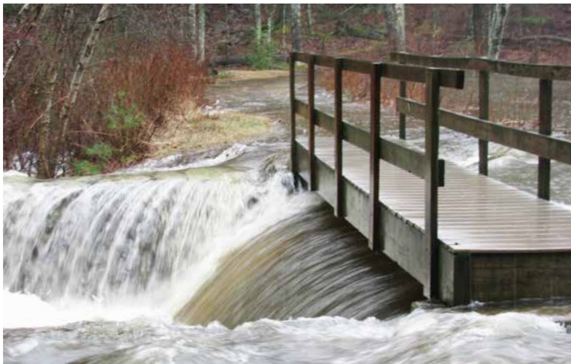
Like many areas across Rhode Island, Audubon's Fisherville Brook Wildlife Refuge in Exeter experienced severe flooding during the spring of 2010. However, the resiliency of the property helped to mitigate even greater damage that could have occurred nearby. Flooded pond crossing shown above.
