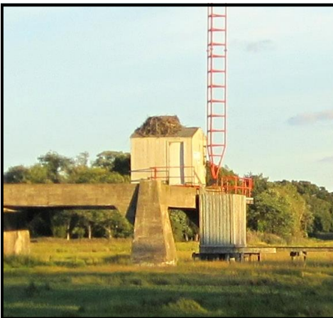
Photo 23: Barrington WPRO radio tower. Photo by Virginia Brown
