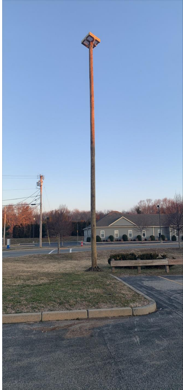
The newly installed QDC nest pole, 2024. Photo by Bill Howard.
