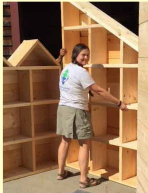
Insect hotel under construction
