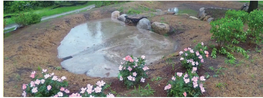
Green infrastructure installments, like the one shown above in Roger Williams Park, reduce stormwater contaminants from entering ponds and degrading water quality.
