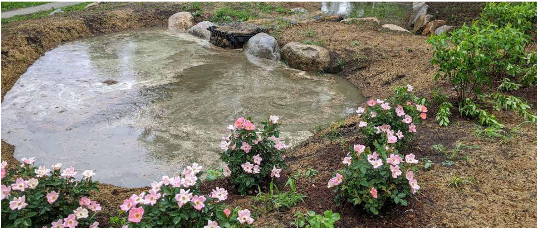
This infiltration basin, built in 2019, is designed to reduce phosphorous loads by 11.6 lbs/year rather than being discharged directly to the ponds at Roger Williams Park.
