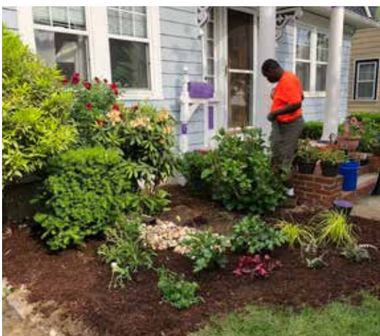
The Woonasquatucket River Watershed Council worked with homeowners in Elmhurst for stormwater retrofits, including redirecting roof downspouts away from the road and toward existing landscaping, installation of permeable pavers in place of walkways, and construction of rain gardens.
